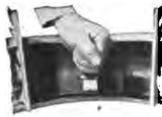
Then cut a third layer (Para coated both sides) 1" larger, and place over second layer in same manner and roll it down.
